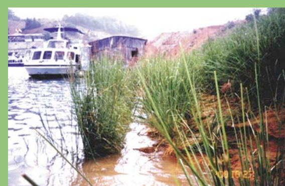
China - partially submerged vetiver grass used to stabilize the draw-down slope of a reservoir in Guangdong Province
