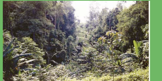
Thailand - a gas pipeline was laid through tropical forest. On steep slopes the right of way was stabilized with vetiver - native plants regenerated
