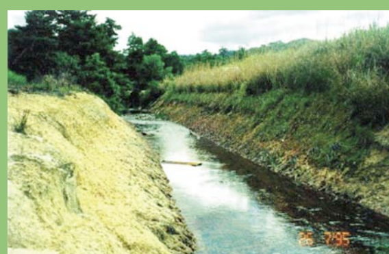
Australia - VS protects the right hand bank of a drain cut through acid sulphate soils of Queensland. Note left hand bank is devoid of any vegetation
