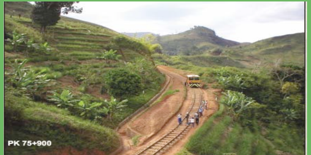
Disaster mitigation - this railroad in Madagascar was closed down by frequent cyclone damage. Stabilization with vetiver was vital in its rehabilitation
