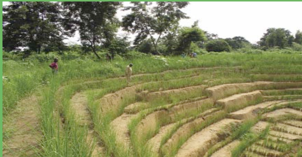
Congo D.R. - huge gullies that destroy urban areas and houses can be rehabilitated and stabilized using the Vetiver System.
