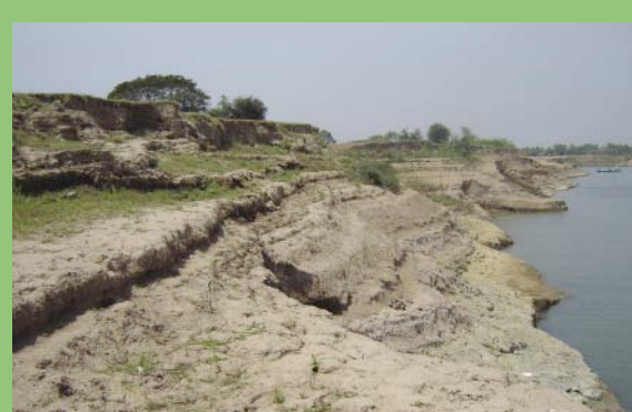
Cambodia - This very large bank on the Mekong River has been under continuous erosion. The land owner with assistance from TVNI is stabilizing using vetiver hedgerows.
