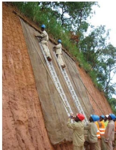
ABOVE: An almost vertical slope being clad with BioJute. Safety is always meticulously taken into account on Rio Tinto's projects.
