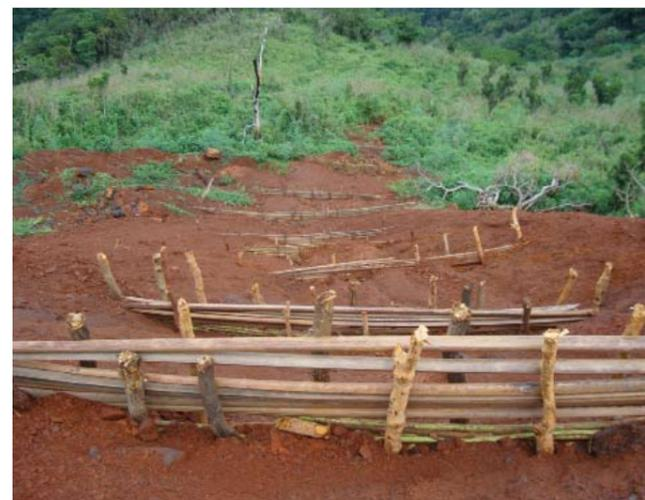
ABOVE: Palm fronds were collected to build 'trash bunds' for soil retention on the steep slopes.
